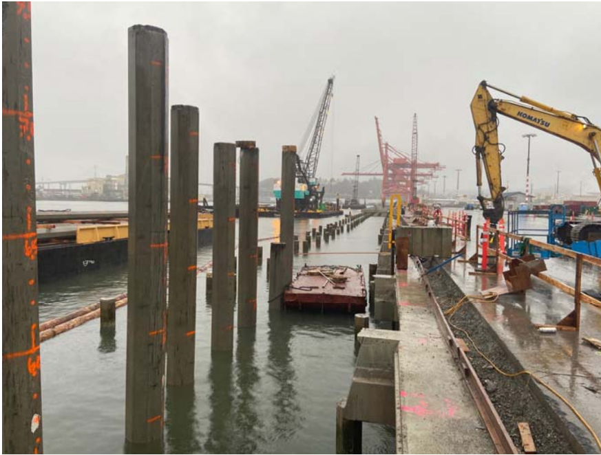
Concrete Pile Installation
