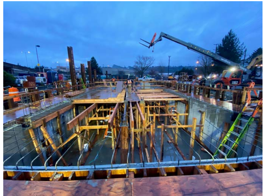
Primary Substation Floating Floor
